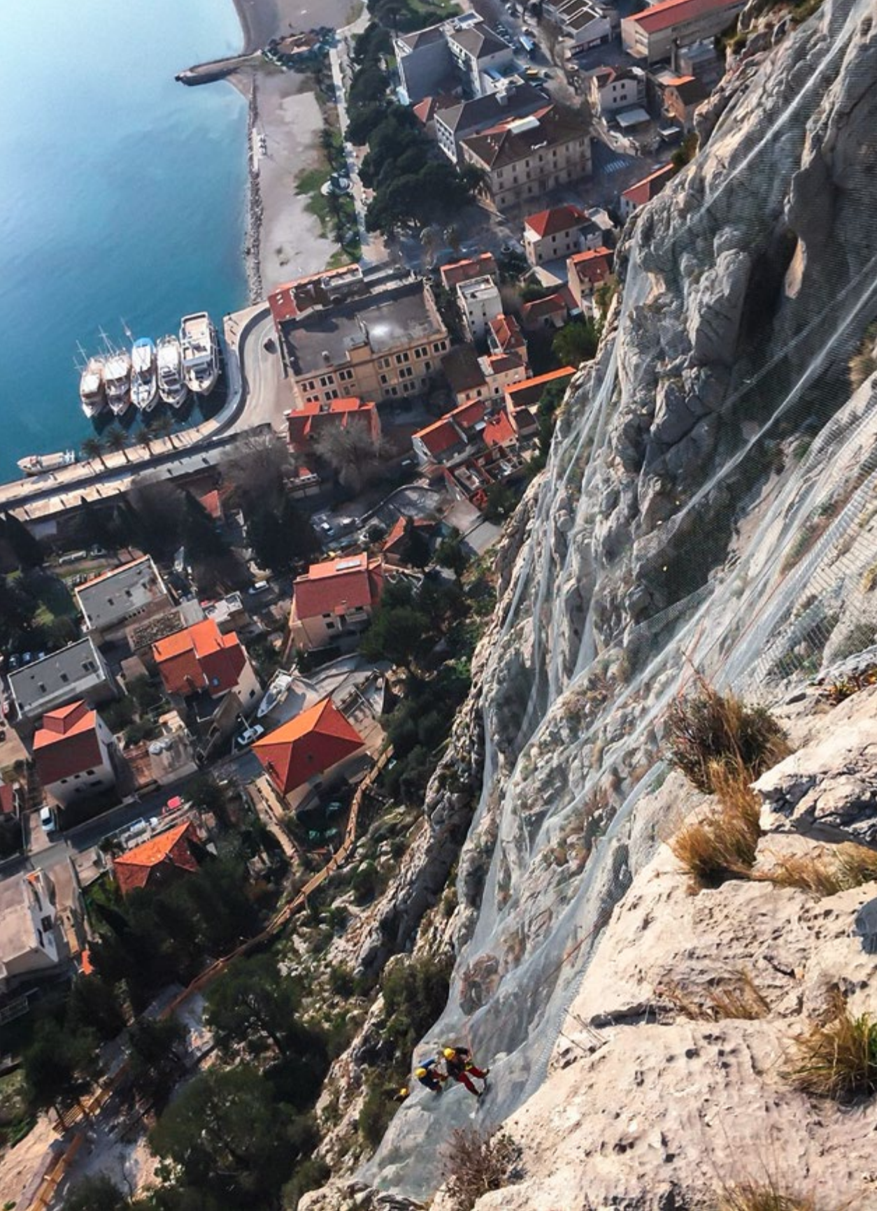
Croatia, Omiš: construction of rockfall protection and rock networking
