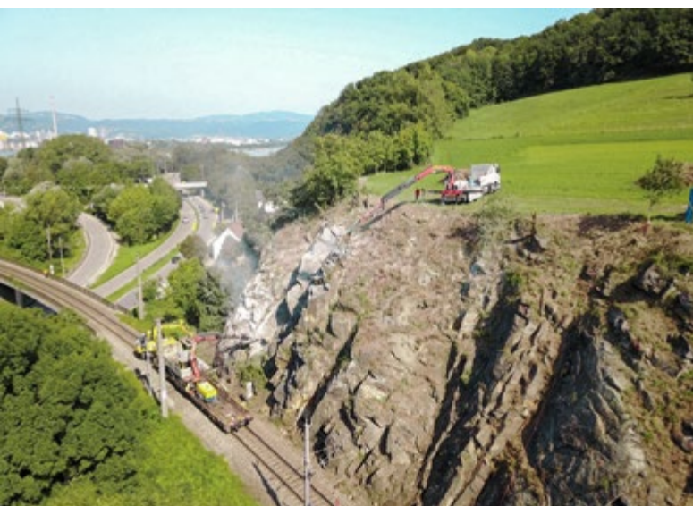
Austria, Steyregg: clearing and slope stabilisation
